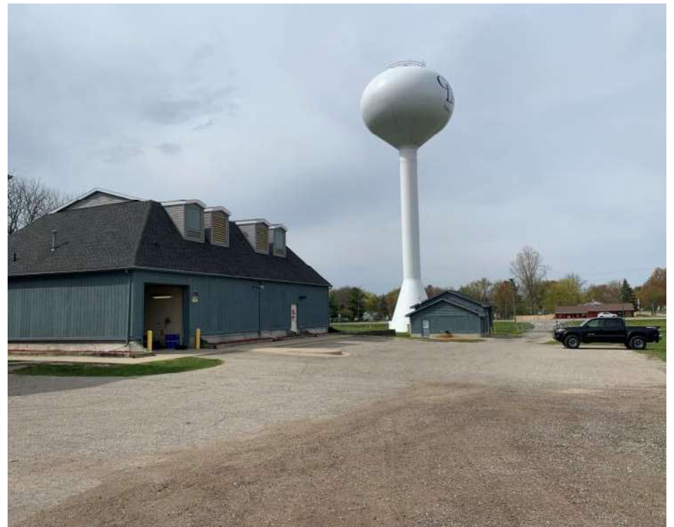
Existing Iron Removal Plant Site
