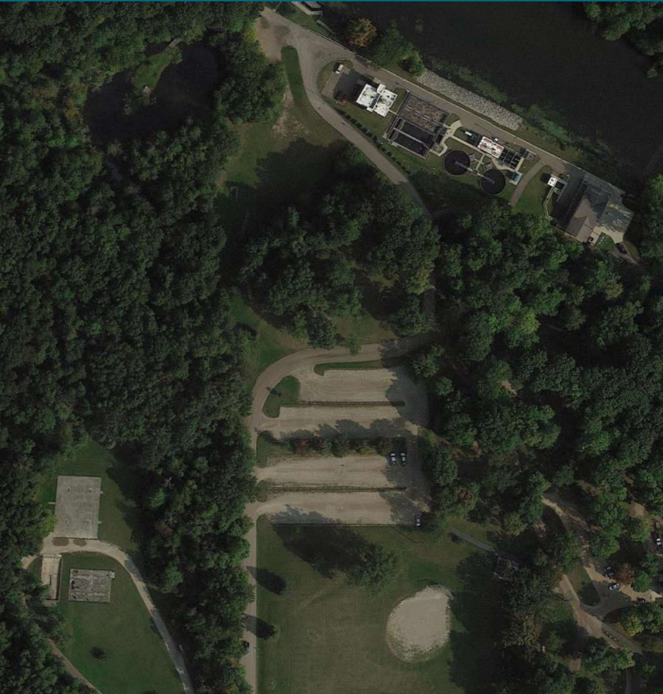
Aerial View of Existing WWTP
