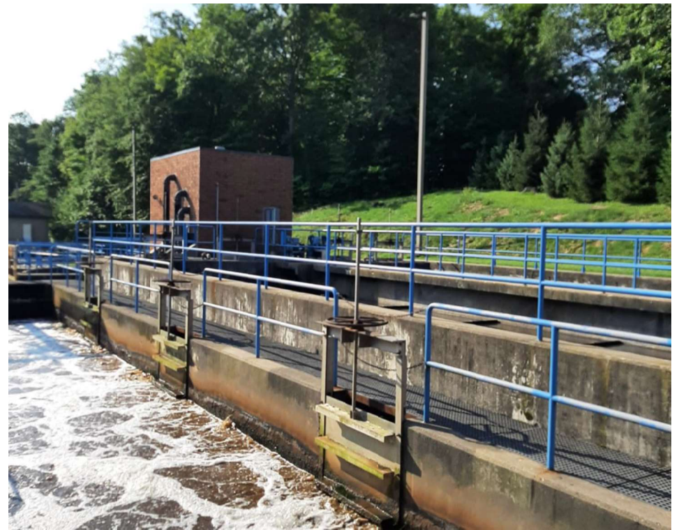
Existing Aeration Tanks
