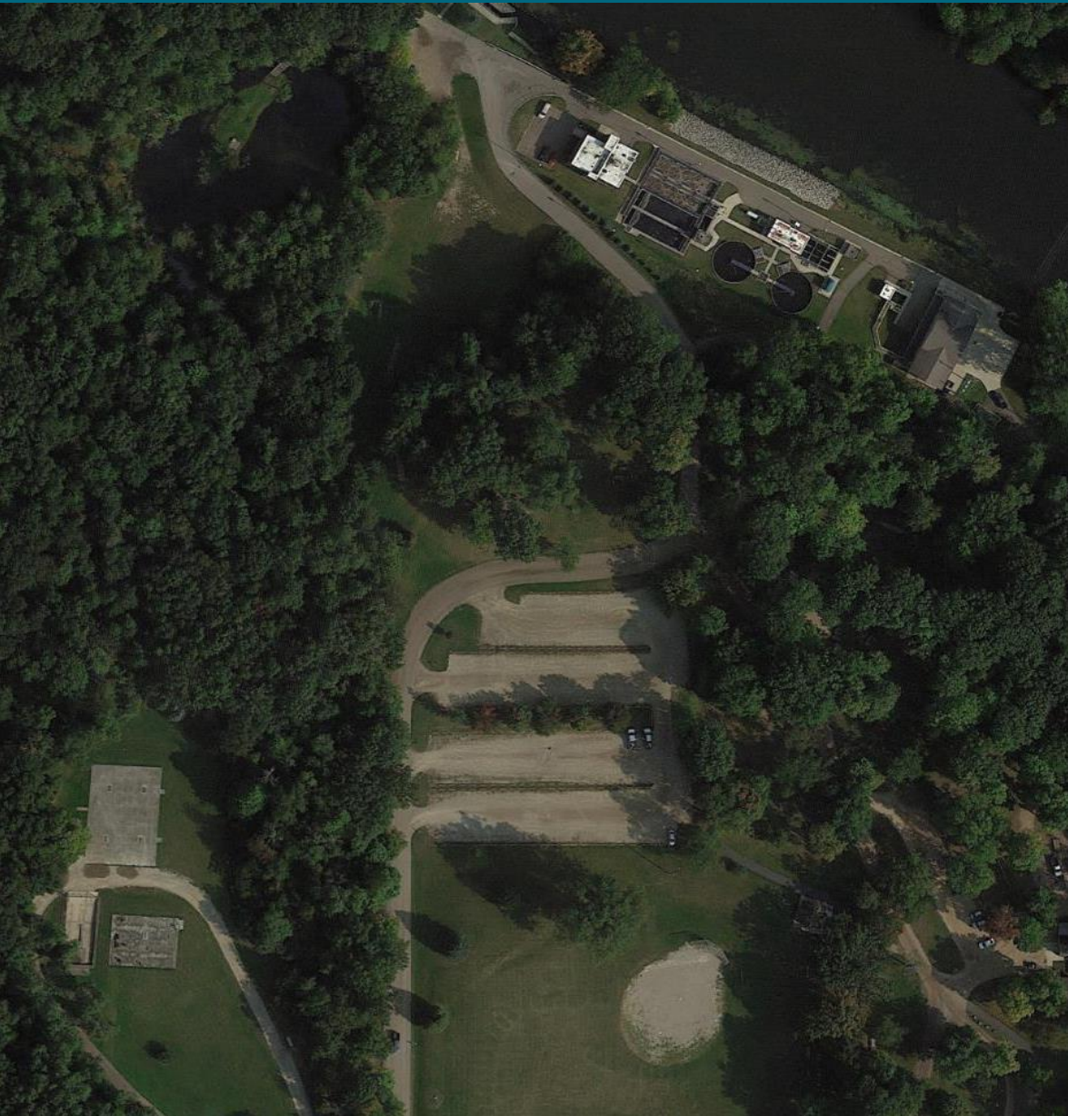
Aerial View of Existing WWTP
