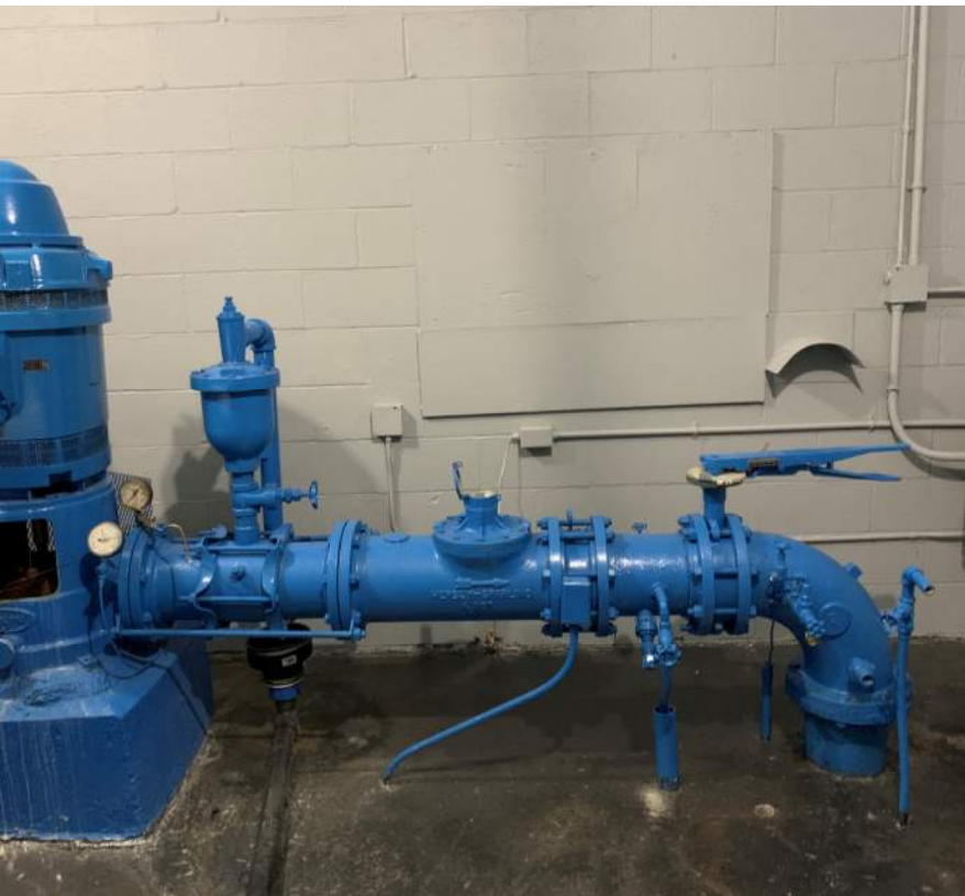
Interior of Wellhouse No. 6
