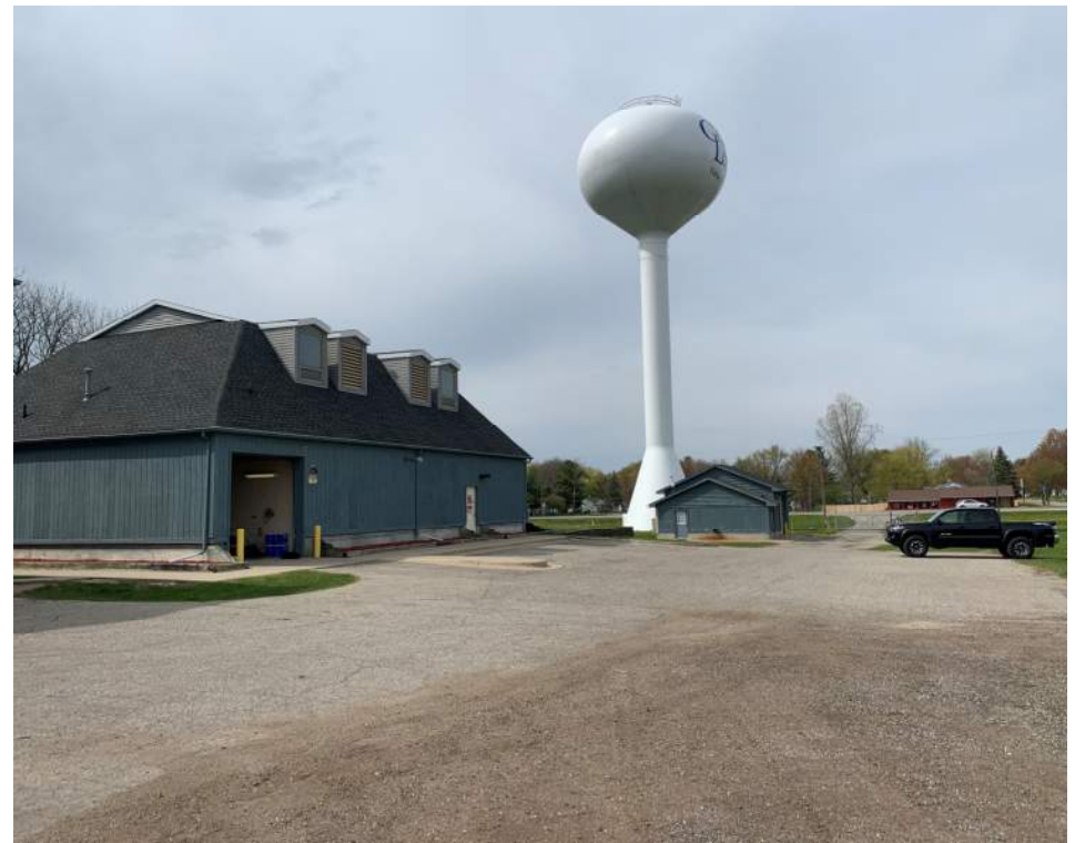
Existing Iron Removal Plant Site
