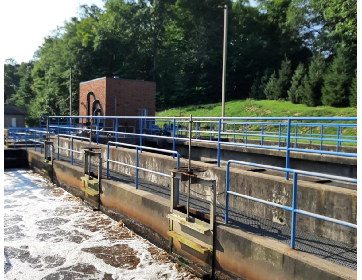
Existing Aeration Tanks
