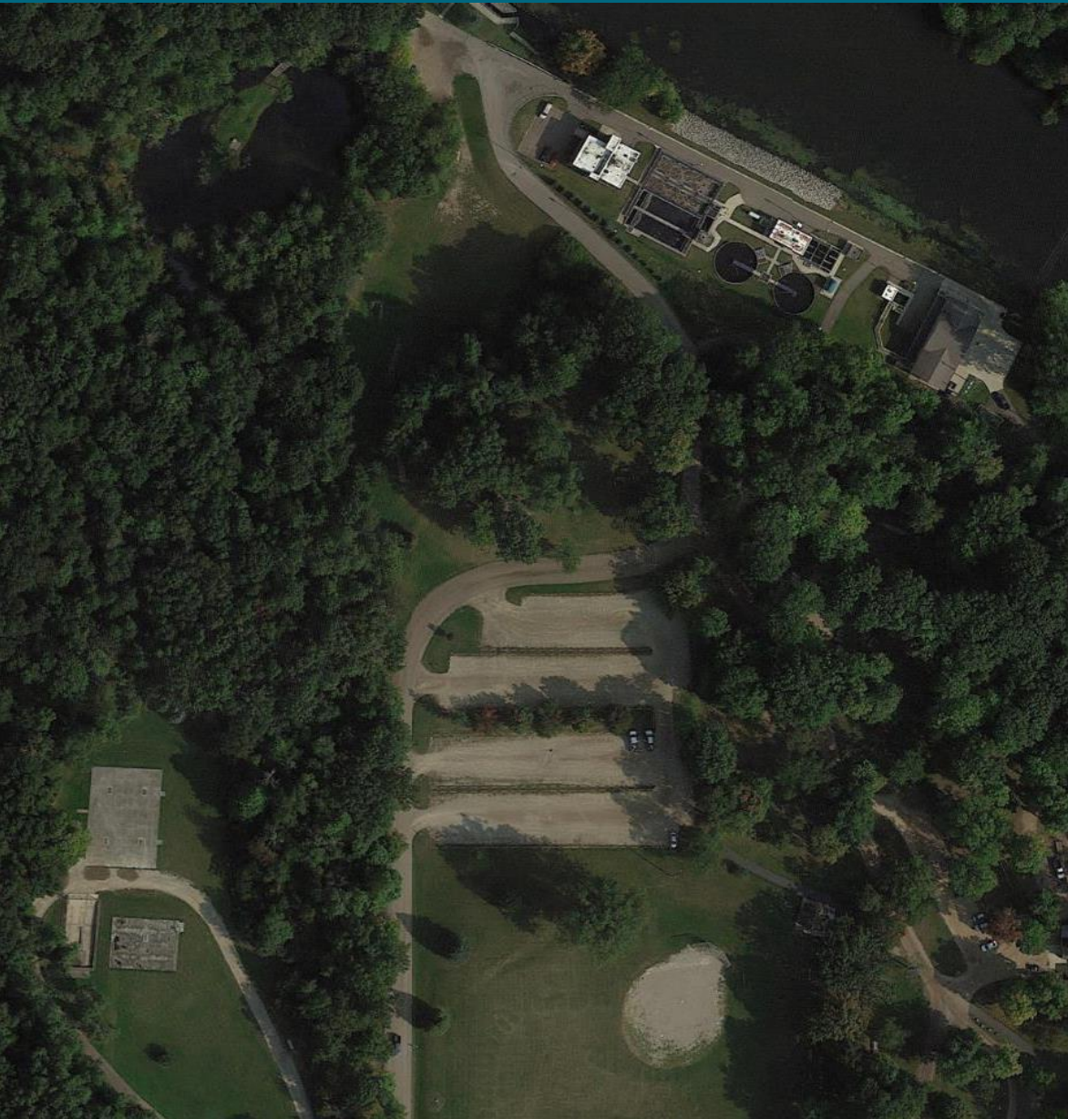
Aerial View of Existing WWTP
