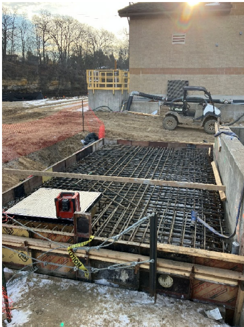
Valve Vault Lid Resteel
