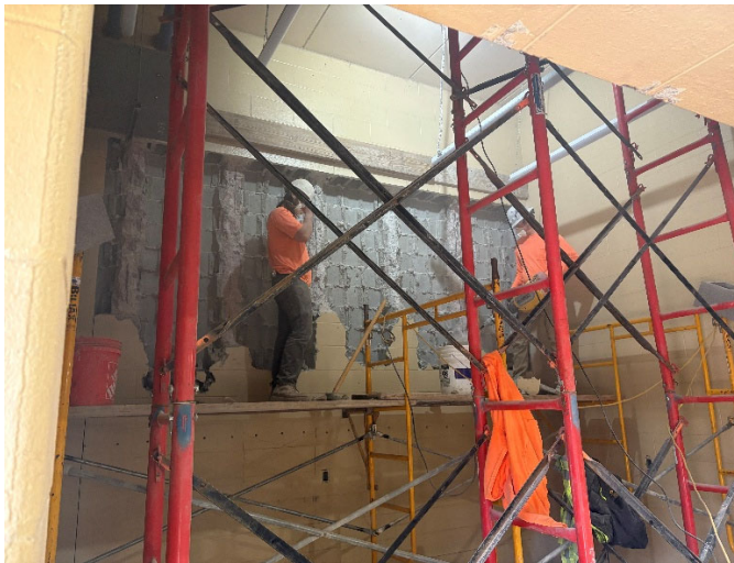
Headworks Building Block Removal
