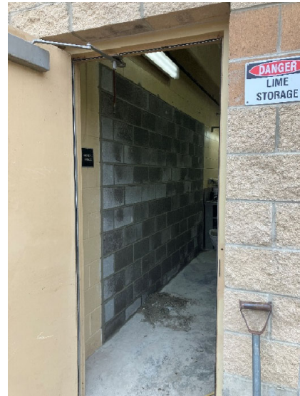
New Headworks Wall
