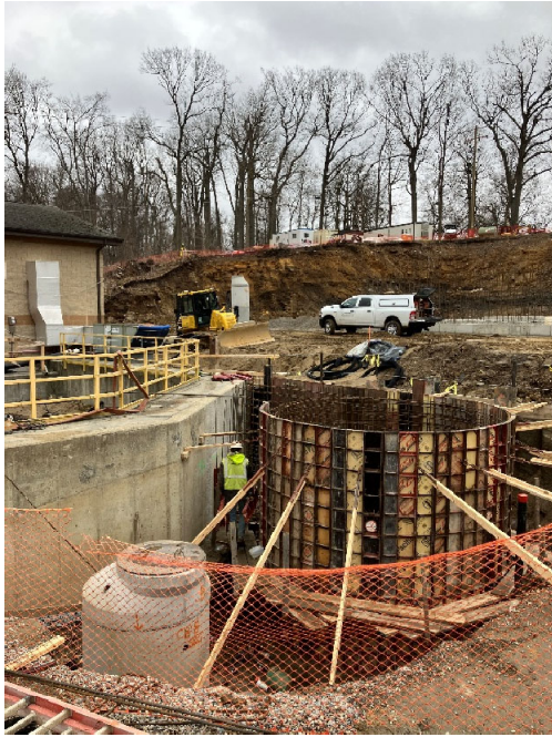
Vortex Grit Tank Forms
