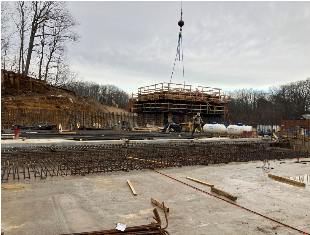
Tank Base Slab And The Start Of Resteel Installation
