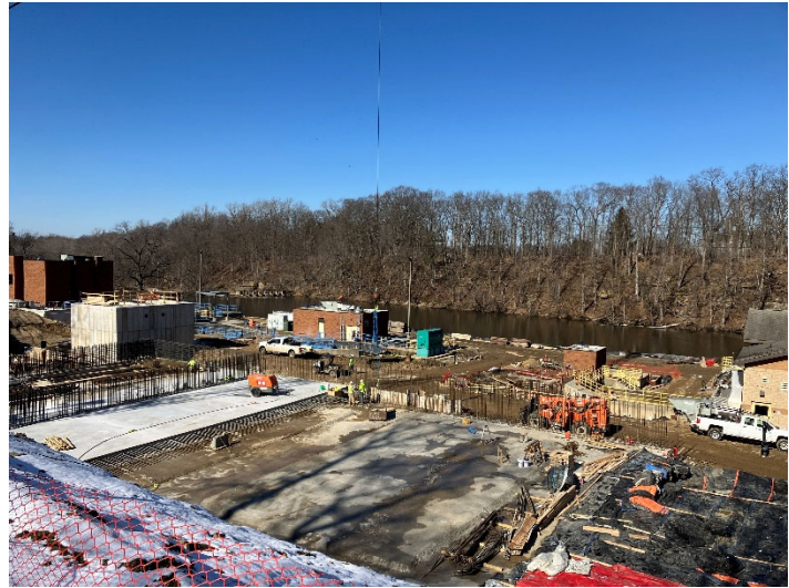
Construction Site Overview
