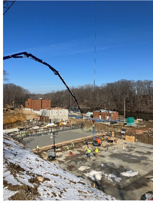
Concrete Pumping For Tank Floor
