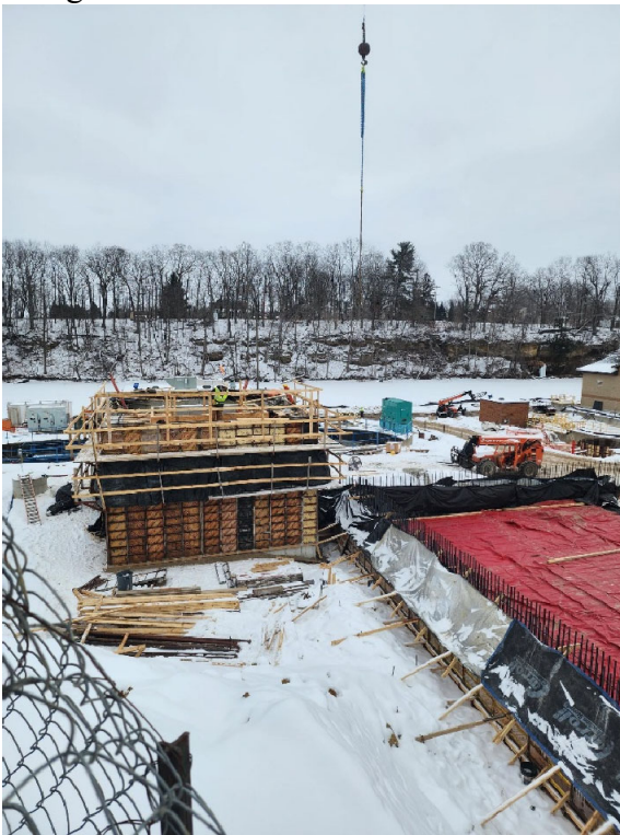
Sludge Buffer Tank walls
