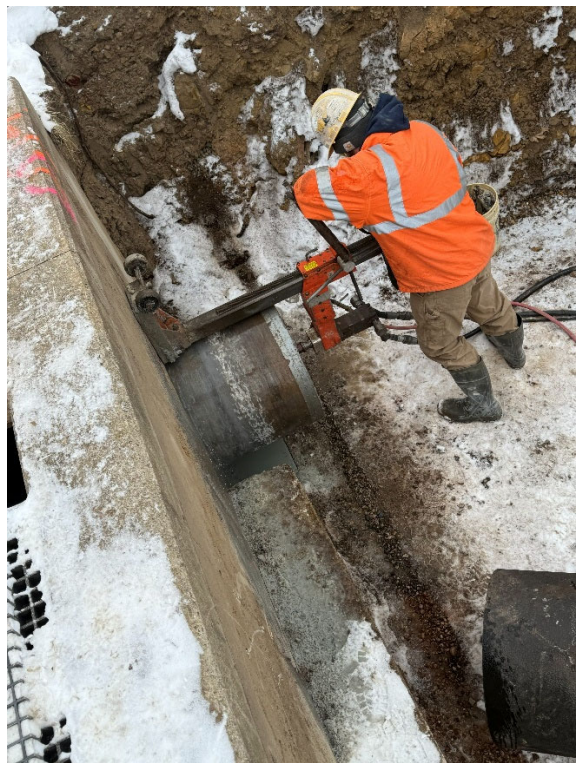
Diversion Structure hole core
