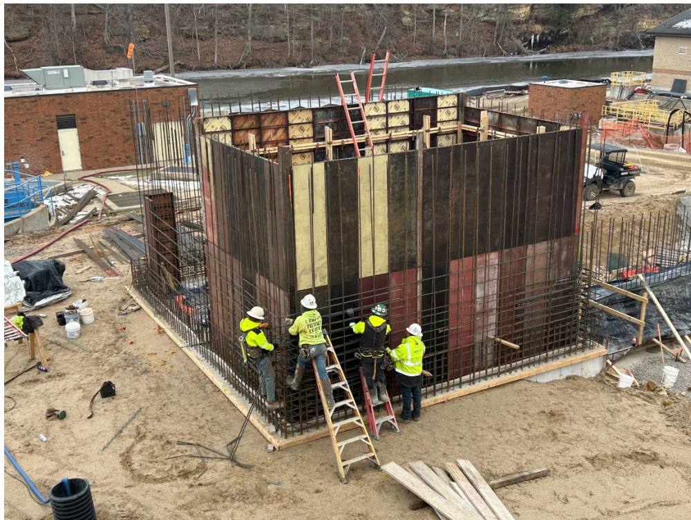
Solids Buffer Tank Forms
