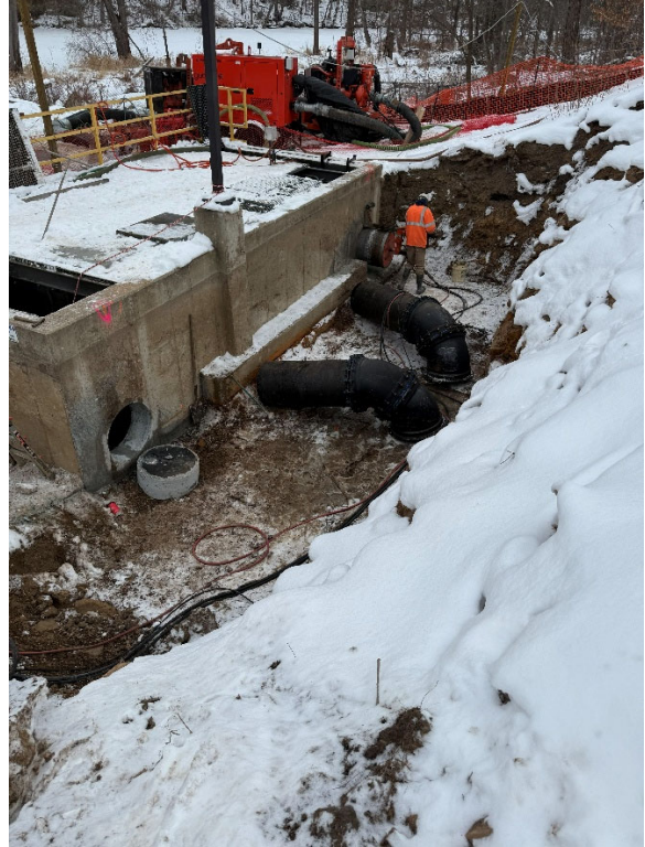
Diversion Structure hole core
