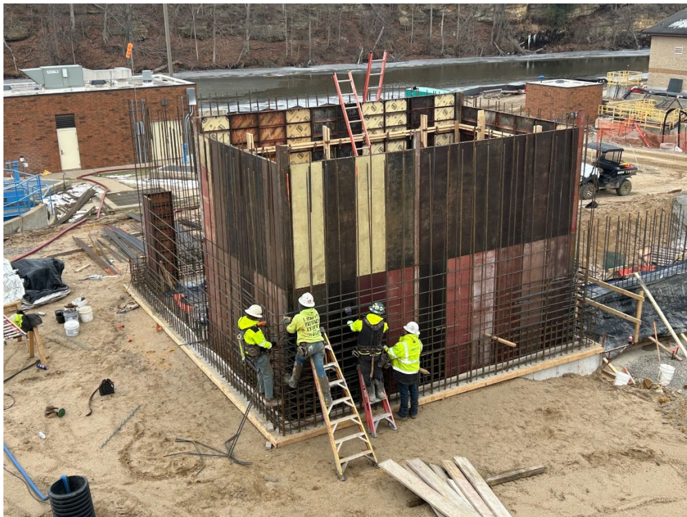
Solids Buffer Tank Forms
